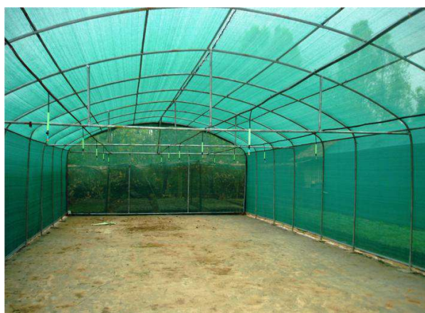
Fig.3. Sprinkler irrigation system in a shade net nursery.
