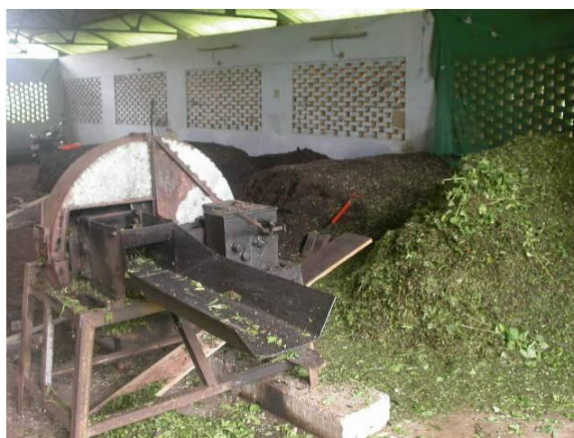
Fig.1. Composting unit showing a well ventilated hall and a weed chopping machine.
